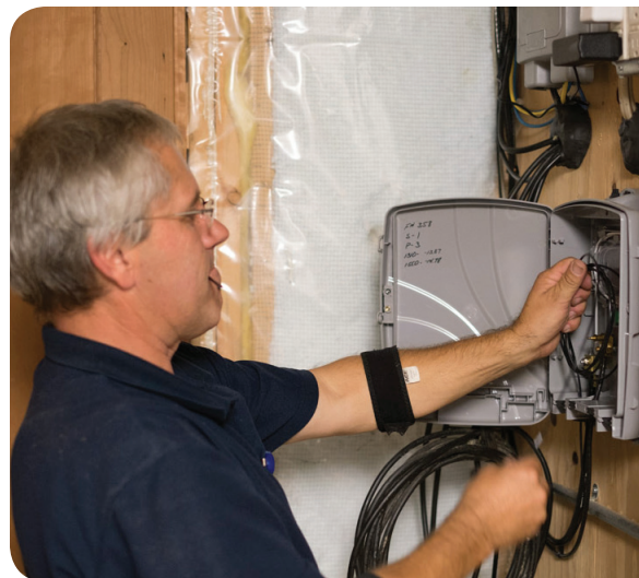
CTC installing a network ONT at the customer premise.
